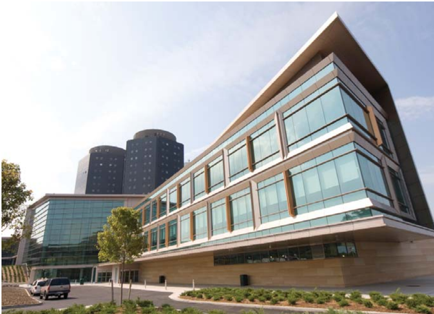
Newly constructed entrance to Stony Brook University Medical Center, part of ongoing modernization.
